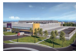
Virginia Ashburn 4 Data Center
