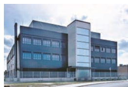
Germany Frankfurt 4 Data Center
